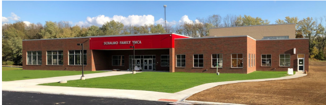
Schalmo Family YMCA Facility
